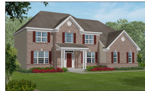
19 Parkside Drive Spec Home Under Construction $599,999
