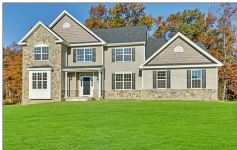
22 Parkside Drive Completed Spec Home $624,900
